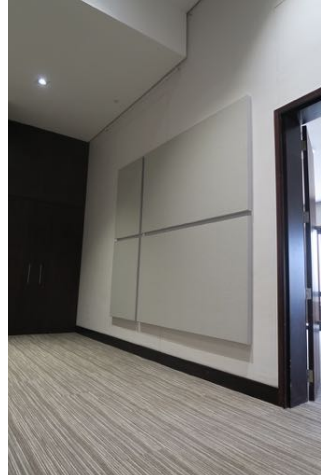
Zimbali Conference Centre - reverberation control Design and Manufacture of Acoustic panels and custom brackets
